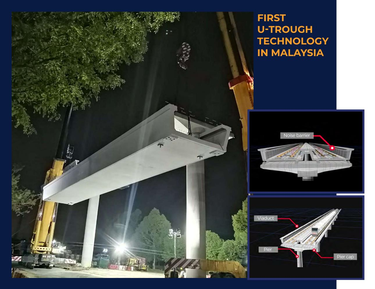
Another first was MRCB's use of innovative U-Trough Girder technology, which allowed construction components to be pre-fabricated, a method known worldwide for being efficient and cost-effective. This was the first project in Malaysia to utilise this groundbreaking technology, which not only puts Malaysia on the global map of infrastructure innovation but also sets a new standard for future railway projects in the country.
