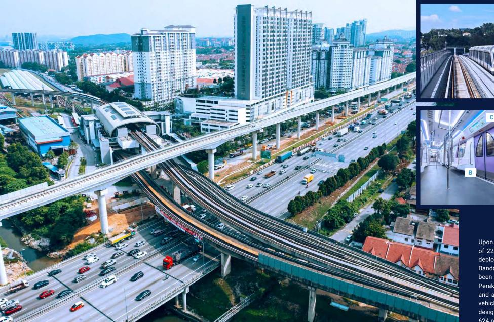
The project's long-span structures, a significant feature of the LRT Shah Alam Line, were strategically designed to optimise the alignment and minimise the number of piers required. The successful completion of 17 long-span structures, varying from 35m to 108m, are seamlessly integrated with U-trough girders employing advanced engineering techniques, ensuring the structural integrity and durability of these longspan structures.
